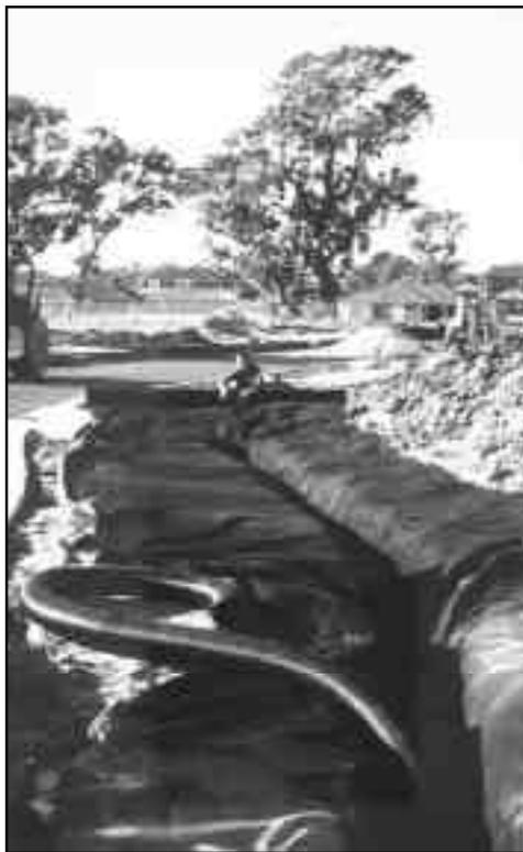
Photo 5: Geotextile placed
