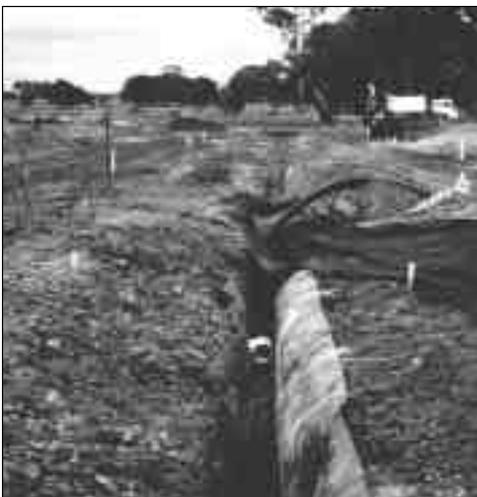
Photo 2: Construction of gravel trench
