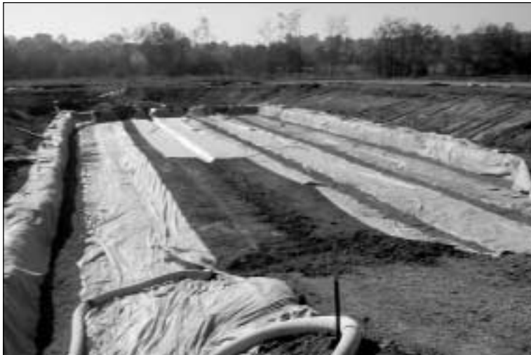
Bioretention system being constructed for stormwater treatment in Brisbane.
