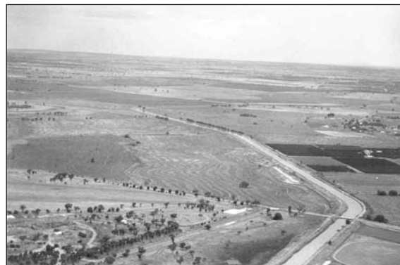
Aerial view of the Leeton irrigation canal
