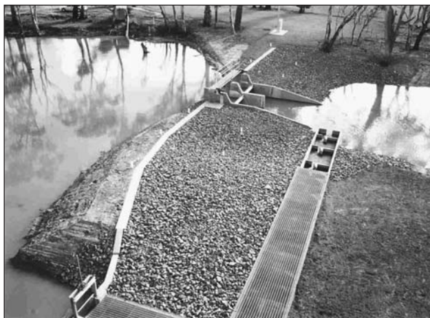
Fishway incorporated into a replacement weir on Broken Creek
